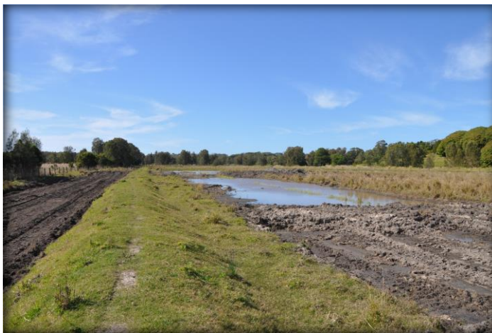
Plate 4.3 Grassed Bunding to 1.8m AHD (formed September 2016) (Photo E617G_048)
