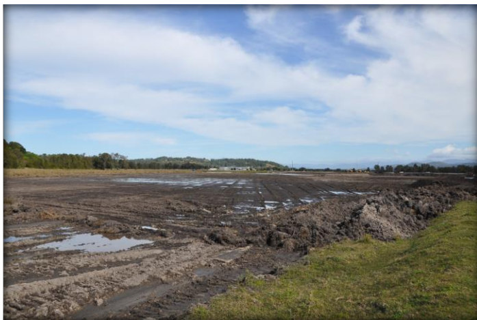
Plate 4.4 Stage 1 Extraction Area & Extension to Bunding (right) In Progress (Photo E617G_069))
