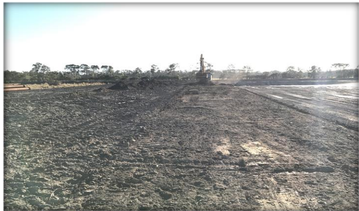
Plate 4.3 Soil Stripping Operations
