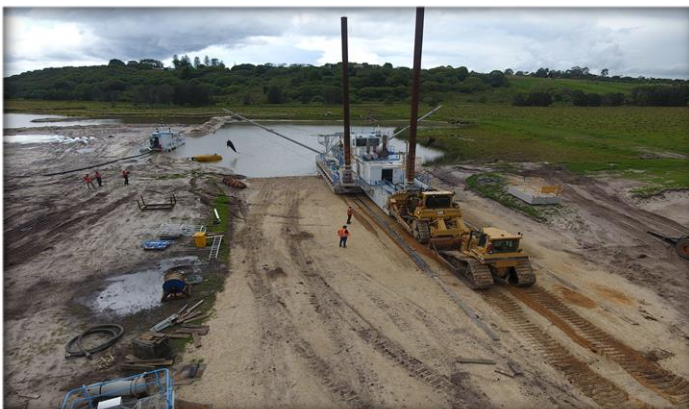
Plate 4.4 Launch of Cutter/Section Dredge
