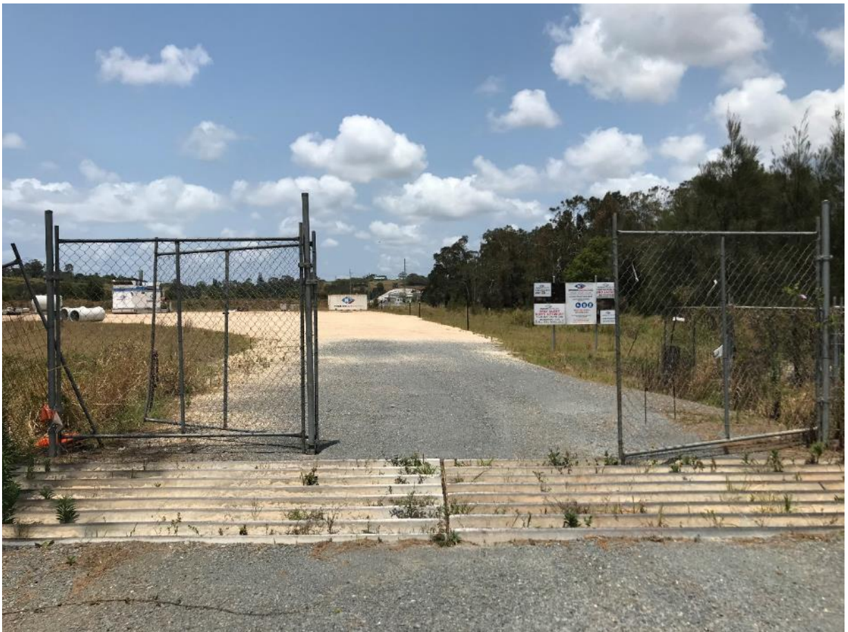
Photo 2. Site access/egress gate with rumble grid installed.
