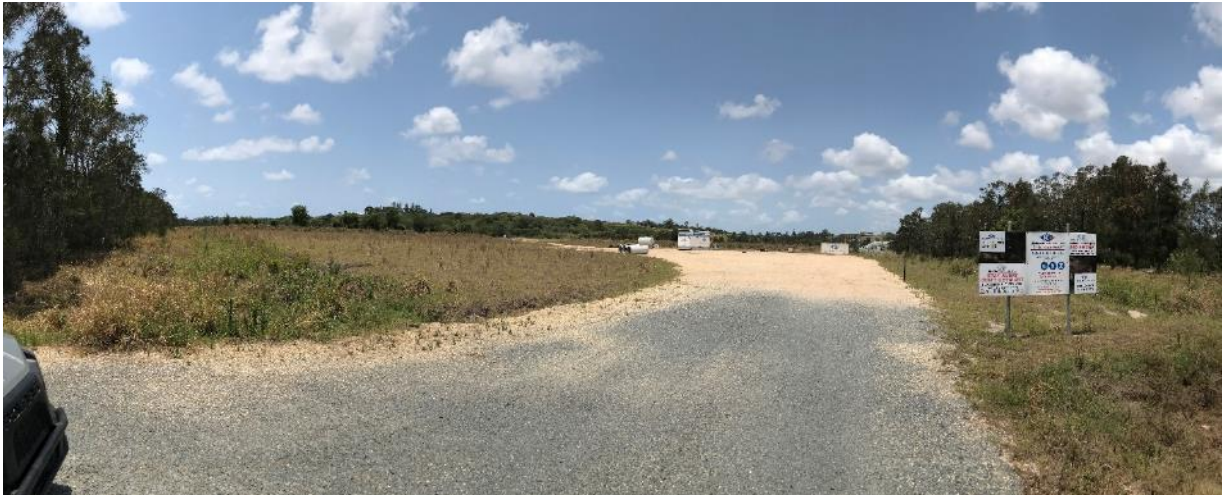
Photo 1. Panoramic view of the site from the entry. No operations at the site during this audit.
