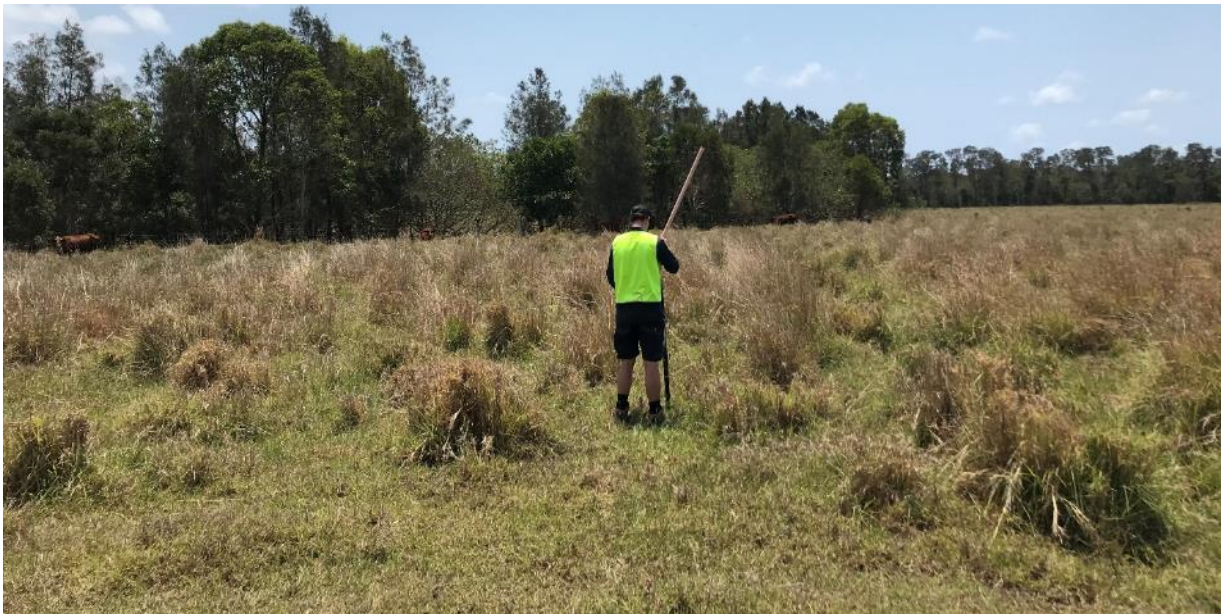
Photo 4. Boundary markers (2 metres peg) were installed around the perimeter of the site.
