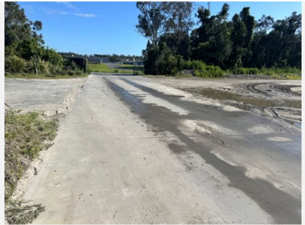
Concreted road to site exit
