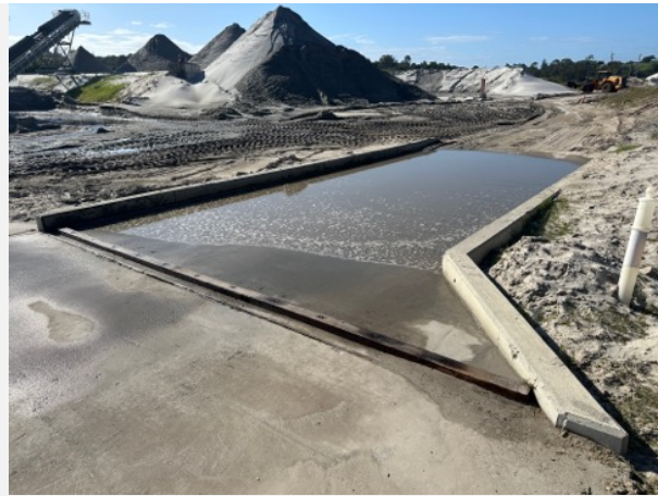
Wheel wash and rumble pad.
