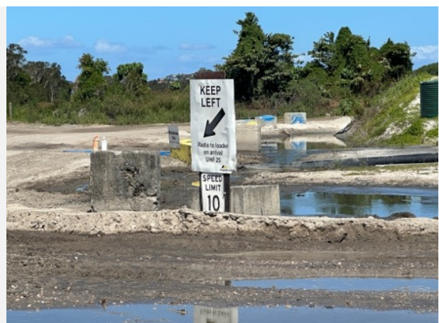
Site speed limit sign
